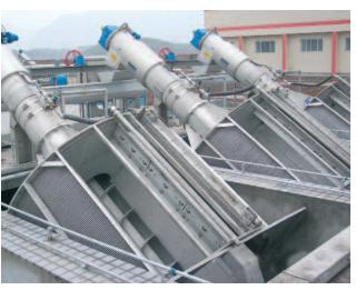
Several parallel ROTAMAT® Fine Screens installed in the channel
