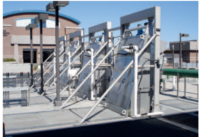
Four STEP SCREEN® SSV: L= 5300, W=1376, 6 mm slot width, installation angle 75°. Maximum operational stability due to the special bottom step design for increased operational reliability without impairment by grit, gravel and stones.
