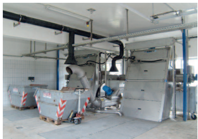
Two STEP SCREEN® Vertical SSV, length 4300 mm, width 1676, 6 mm slot width, combined with HUBER Wash Press type SL for intensive screenings washing. Totally enclosed, odour-free design.
