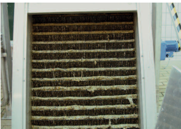
STEP SCREEN® Vertical SSV: very high separation capacity due to the fine slot widths and the produced screenings carpet.
