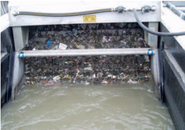
STEP SCREEN® Flexible SSF: length 3500, width 1826, slot width 6 mm, installation angle 50 °, high capacity as the flow passes the screen surface only once.
