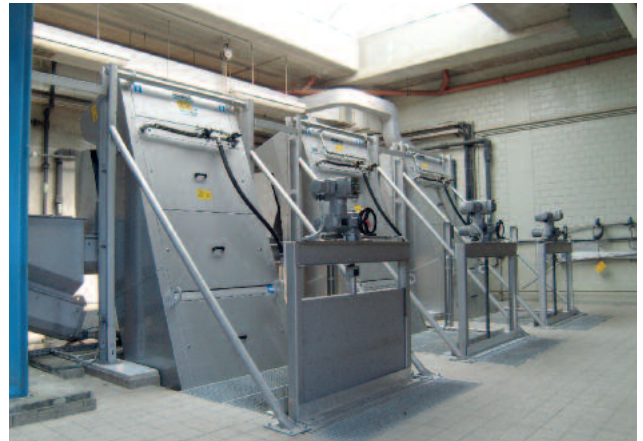
STEP SCREEN® Vertical SSV: 4300 mm long, 3 mm slot width, acid treated in a pickling bath for optimal corrosion protection
