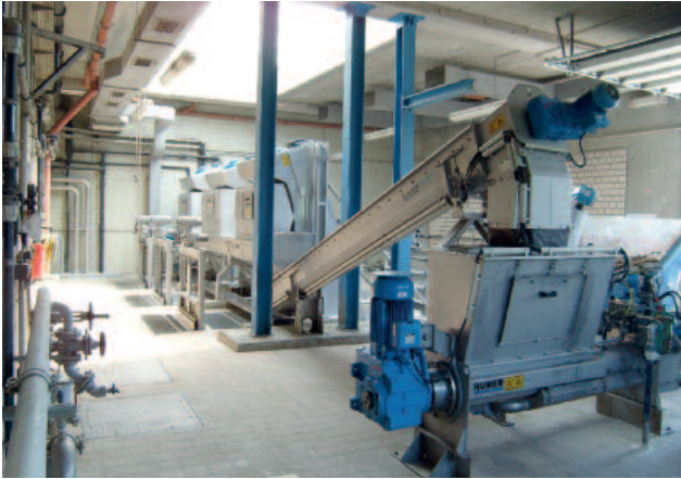
3 STEP SCREEN® Vertical SSV units: length 4300, width 1176, slot width 3 mm. Optimally adjustable to suit specific constructional conditions (big discharge height, deep channel) due to the steep installation angle of 70° to 80°
