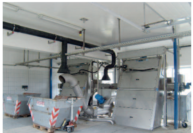
2 STEP SCREEN® Vertical SSV, length 4300 mm, width 1676, 6 mm slot width, combined with HUBER Wash Press type SL for intensive screenings washing. Totally enclosed, odour-free design.
