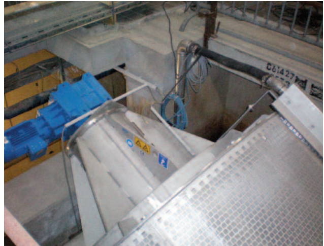
ROTAMAT® Membrane Screen liquid with screenings discharge by pump
