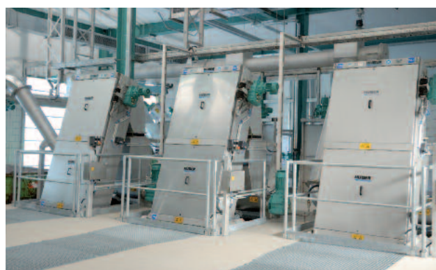
Reliable, sturdy travelling RakeMax ® screen
