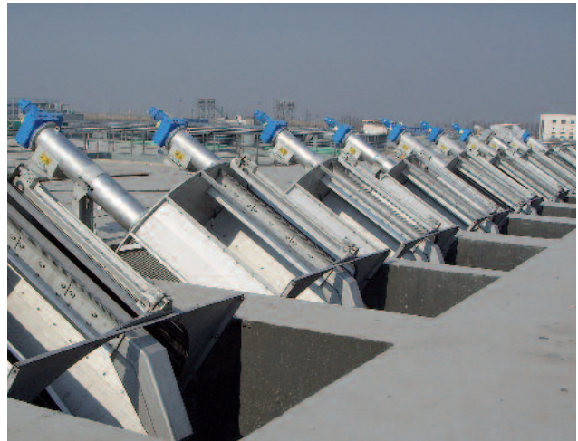
ROTAMAT® Fine Screen Ro 1 for installation in a channel or container
