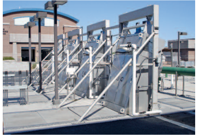
4 STEP SCREEN® SSV units: length 5300, width 1376, slot width 6 mm, installation angle 75°. Maximum operational stability without impairment by grit, gravel and stones due to the special bottom step design.
