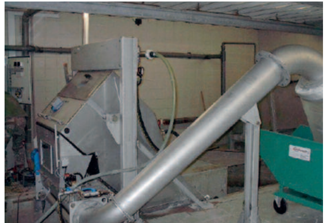
STEP SCREEN® Flexible SSF with HUBER Wash Press for optimal separation and dewatering results. Acid treated in a pickling bath for corrosion protection.
