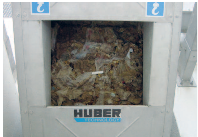
STEP SCREEN® Flexible SSF: very high operational stability and reliable operation without impairment by grit, gravel and stones due to the special bottom step design for lifting of screenings at bottom level.
