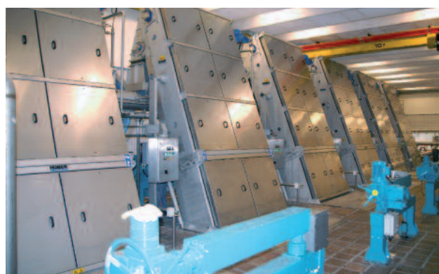
HUBER Belt Screen EscaMax ® – a versatile inlet screen
