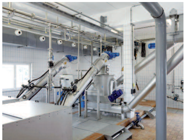
ROTAMAT® Rotary Drum Fine Screen Ro 2 units with closed stainless steel cover
