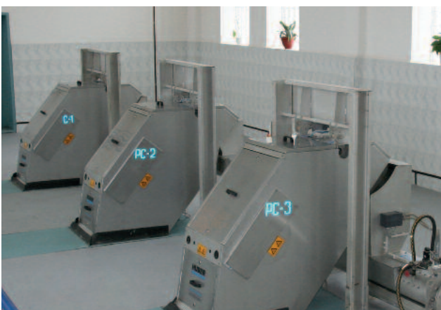
STEP SCREEN® Flexible SSF application in Russia: pivotable in the channel without having to remove the downstream HUBER Wash Press and HUBER Screw Conveyor
