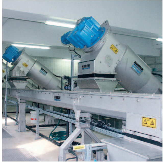
ROTAMAT® Membrane Screen RoMem prior to a hollow fibre membrane plant
