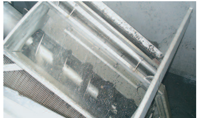
Floating and suspended material is retained in the screen basket. The tines mesh into the basket bars and ensure a complete automatic cleaning.
