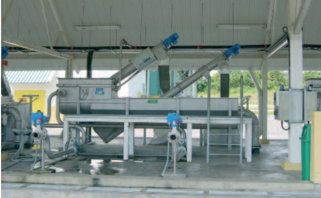
ROTAMAT® Sludge Acceptance Plant with un-aerated grit trap and integrated grit classifying screw
