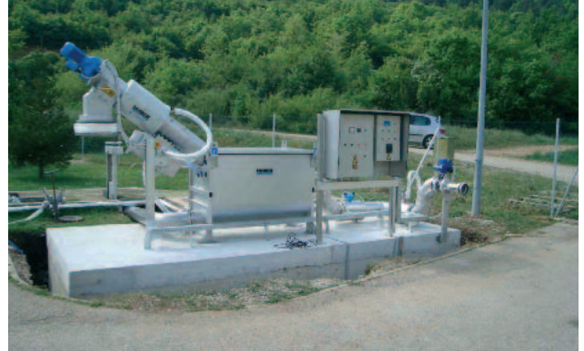
Well-proven mechanical pre-treatment components combined within the ROTAMAT® Sludge Acceptance Plant Ro 3.3
