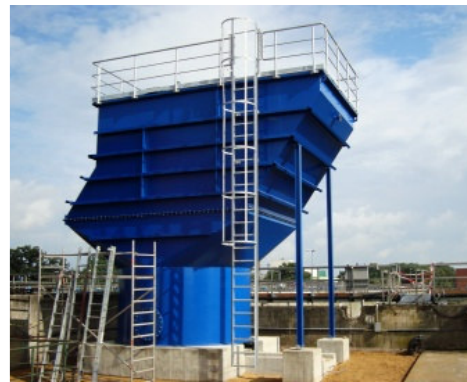
Johnson Lamella separator with 390 m 2 sedimentation area.
