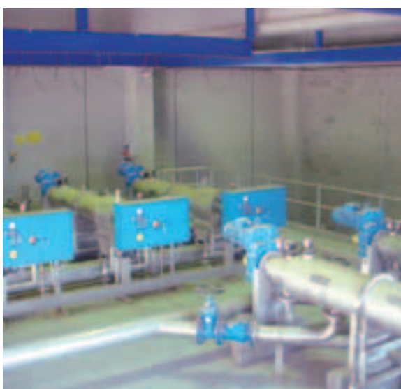
Sludge screening on WWTP Barcelona, Spain
