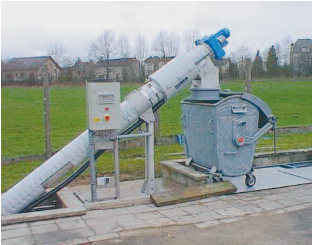
Outdoor installation of a ROTAMAT® Fine Screen Ro 1 with frost-protection
