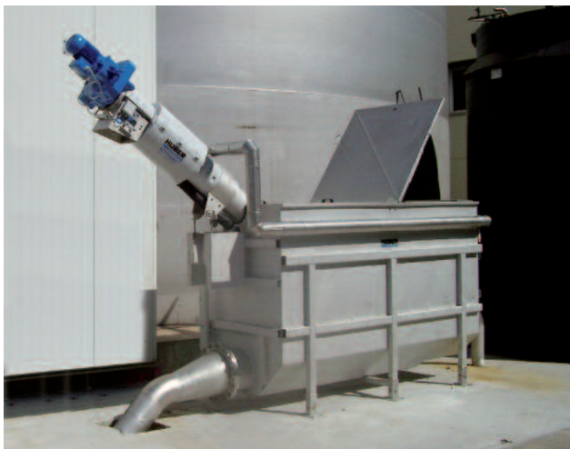
ROTAMAT® Fine Screen Ro 1 in a tank
