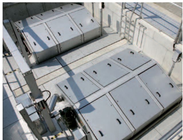
RoDisc® Rotary Mesh Screen for retention of activated sludge flocs
