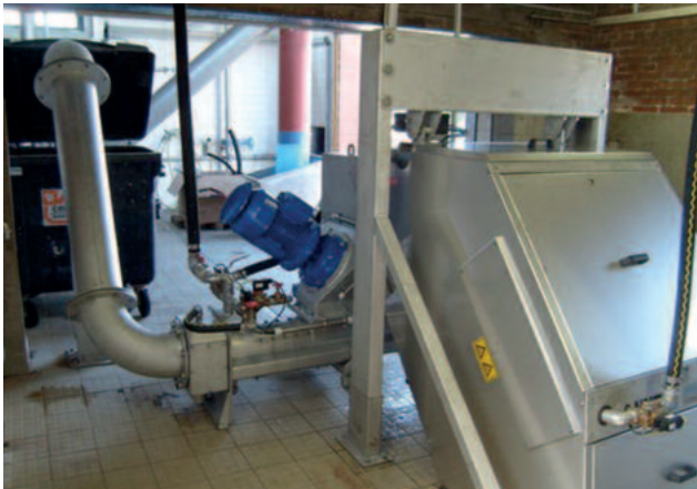
STEP SCREEN® Flexible SSF combined with Wash Press type SL for intensive screenings washing. Totally enclosed, odour-free design.
