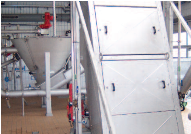
STEP SCREEN® Vertical SSV in channel, pivotable without having to remove the downstream Screenings Wash Press
