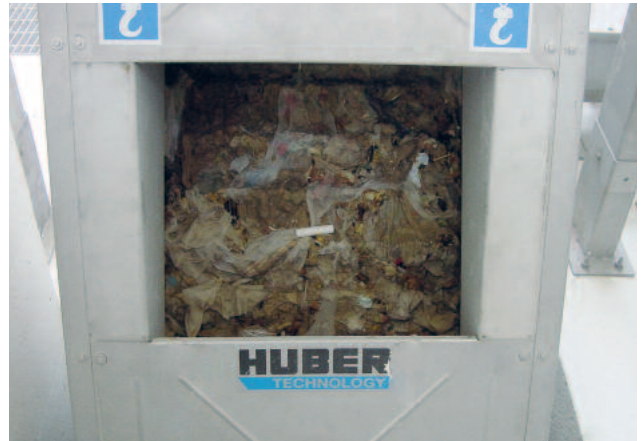
STEP SCREEN® Flexible SSF: very high operational stability and reliable operation without impairment by grit, gravel and stones due to the special bottom step design for lifting of screenings at bottom level.
