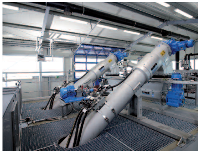
ROTAMAT® RoMem for increased operating reliability of MBR plants
