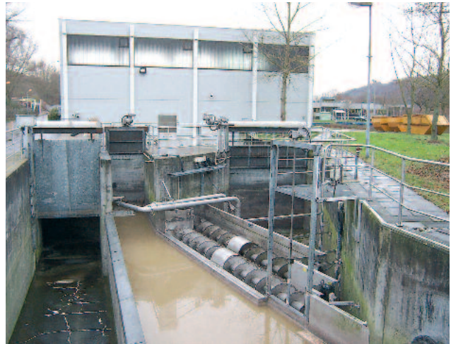
Combination of different screening systems for optimised treatment of large volumes of wastewater
