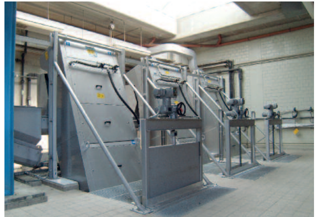
STEP SCREEN® Vertical SSV: 4300 mm long, 3 mm slot width, acid treated in a pickling bath for optimal corrosion protection
