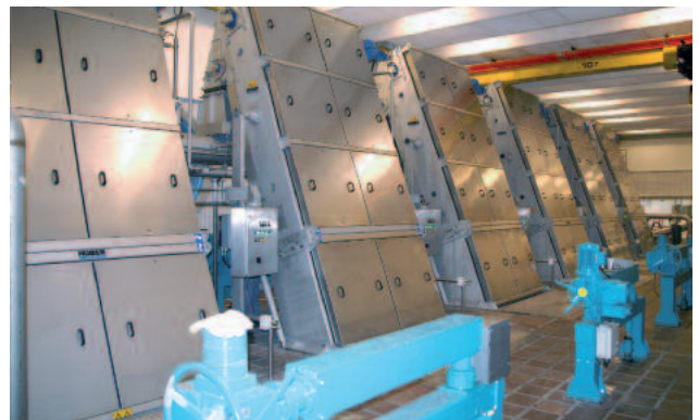
Belt Screen EscaMax® – a versatile inlet screen
