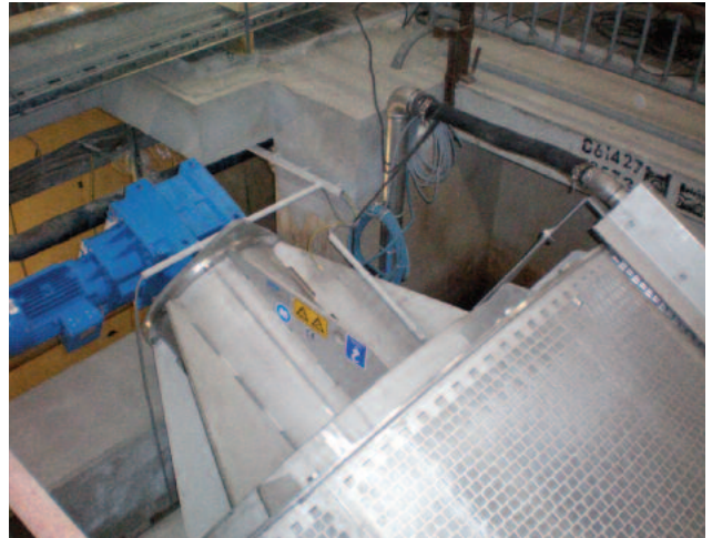
ROTAMAT® Membrane Screen liquid with screenings discharge by pump
