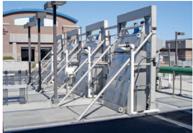
4 STEP SCREEN® SSV units: length 5300, width 1376, slot width 6 mm, installation angle 75°. Maximum operational stability without impairment by grit, gravel and stones due to the special bottom step design.
