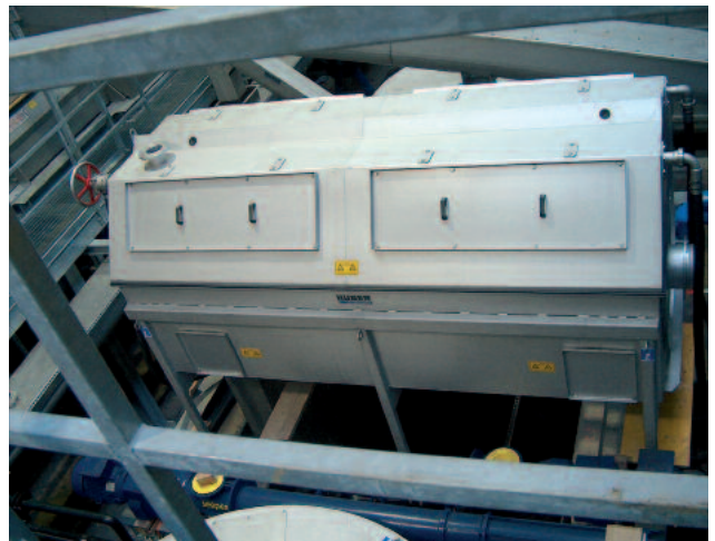
ROTAMAT® Rotary Drum Screen RoMesh® with 0.5 mesh size for wash water recovery
