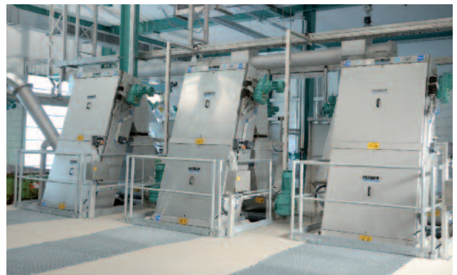
Reliable, sturdy travelling RakeMax® screen
