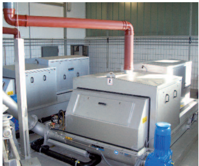
Compact Curved Bar Screen CurveMax® for reliable separation of solids from wastewater
