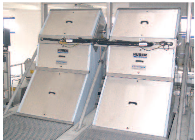
Two STEP SCREEN® Flexible SSF units installed in parallel channels
