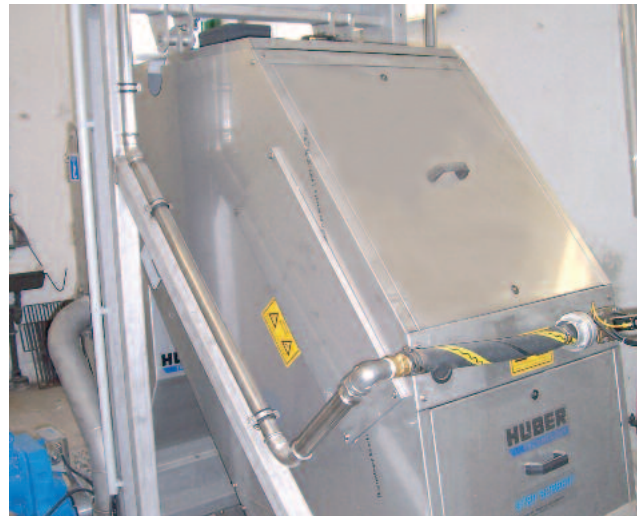
Fully enclosed, odour-free STEP SCREEN® Flexible SSF
