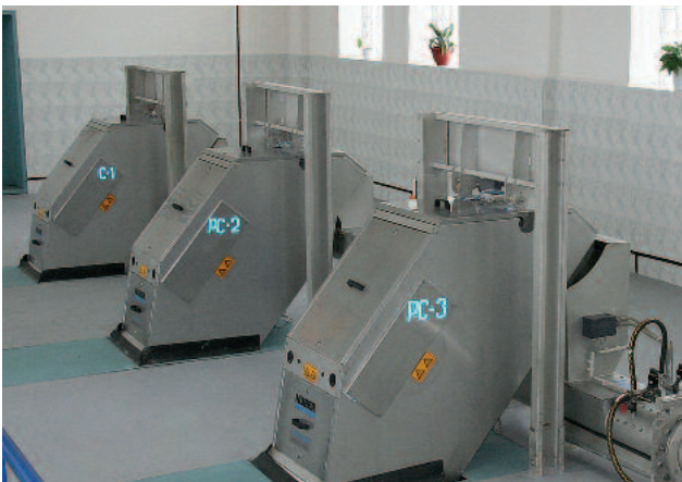
STEP SCREEN® Flexible application in Russia: pivotable in the channel without having to remove the downstream HUBER Wash Press and HUBER Screw Conveyor.
