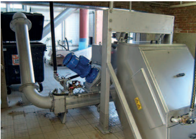
STEP SCREEN® Flexible combined with HUBER Wash Press type SL for intensive screenings washing. Totally enclosed, odour-free design.
