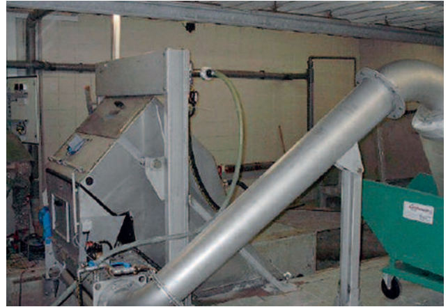
STEP SCREEN® Flexible with HUBER Wash Press for optimal separation and dewatering results. Acid treated in a pickling bath for corrosion protection.
