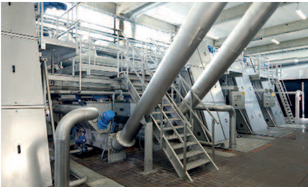
6 HUBER Belt Screen EscaMax® units with HUBER Wash Press WAP-SL: individually adaptable discharge due to flexible launder channel arrangement
