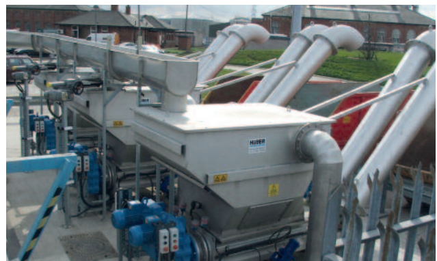
3 HUBER Wash Press WAP-SL units, size 12, maximum throughput 12 m³/h, with launder channel feeding system. Maximum available launder channel length: 40 m.
