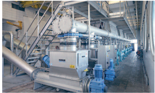
Redundantly operated HUBER Wash Press WAP-SL units with launder channel feeding system. Totally enclosed, odour-free stainless steel design.
