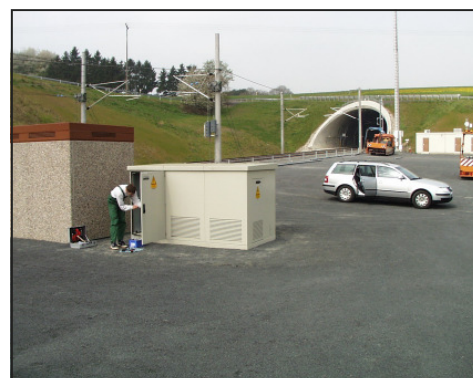
NDV401-train-transformer-substation with 16 \frac{2}{3} Hz
