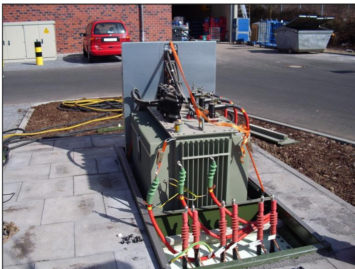
LCS-E, housing detached on-site
