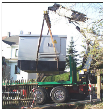
Setting up of a NDV400 by truck-crane
